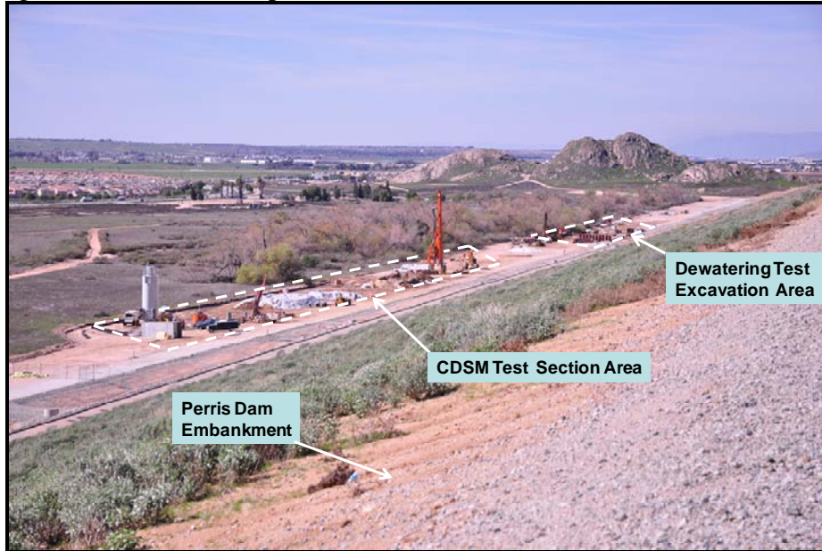
Figure 2. Perris Dam Dewatering Test Excavation and CDSM Test Section
